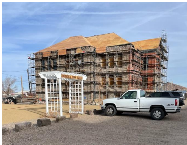
New Plywood Installed
