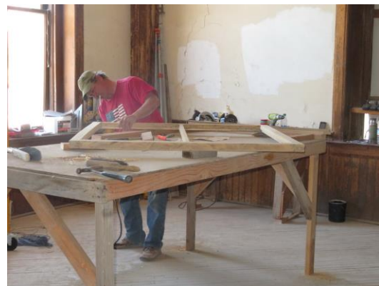
Ron Young working on a window frame
